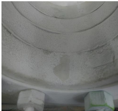
Figure 2.29: Crack observed in the referred wall.
